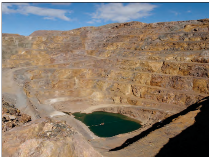
Figure O3. Photograph of the Mountain Pass Mine in San Bernardino County, California, which was the only active producer of rare-earth elements (REEs) in the United States in 2013. The orebody is a tabular carbonatite intrusion and is thought to be the largest REE resource in the United States. Molycorp, Inc. (2012), which owns and operates the mine, reported proven and probable reserves totaling 16.7 million metric tons of carbonatite ore at an average grade of 7.98 percent rare-earth oxide (REO) using a cutoff grade of 5 percent REO. The mine was placed on care-and-maintenance status in 2015. Photograph by Bradley S. Van Gosen.
